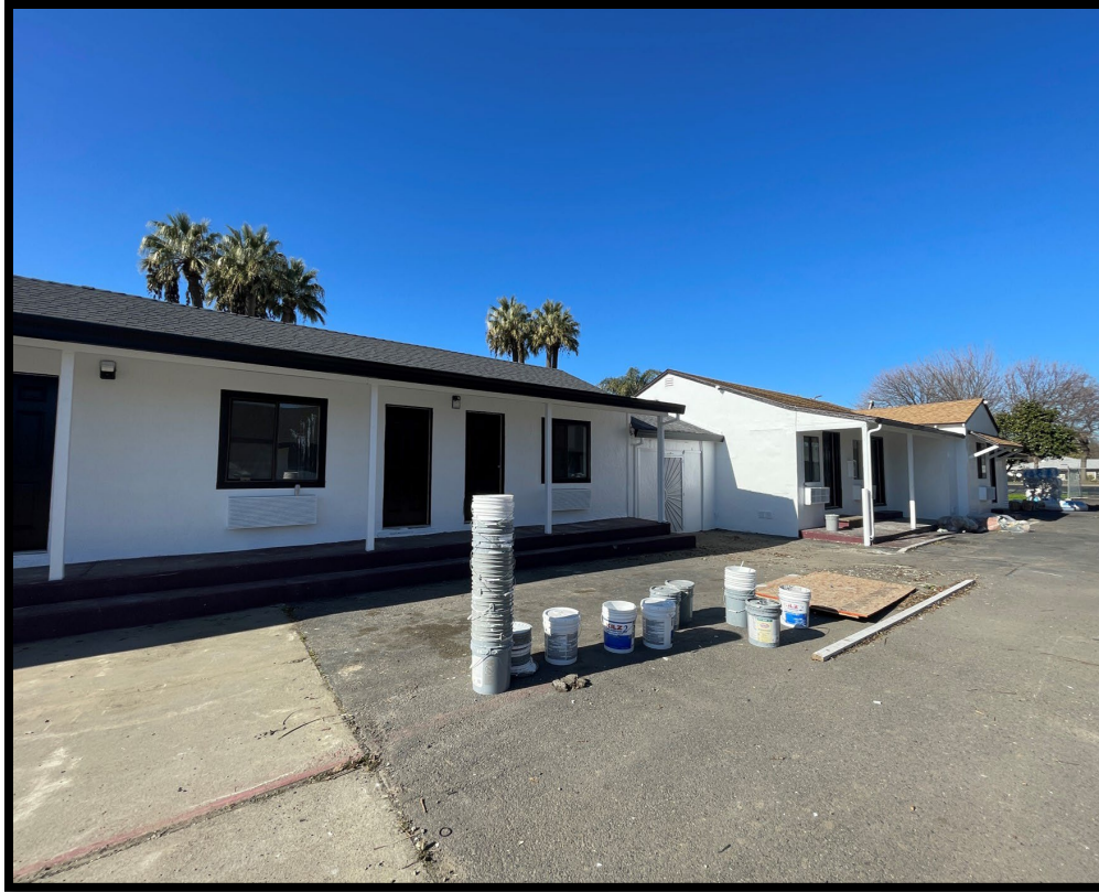
Figure 2 - Emergency Housing Rehabilitation Project – Pickwick Motel
